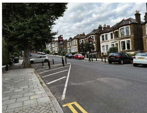
Avoid Avoid hatching and consider how excess space may be used for planting, cycle parking, footway widening or street furniture.
